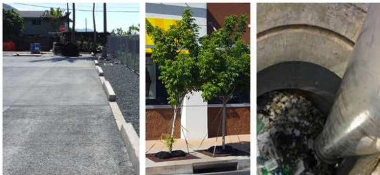
Permeable pavement, tree filter boxes and hydrodynamic separators are examples of Post-Construction BMPs commonly used in Waikiki.
