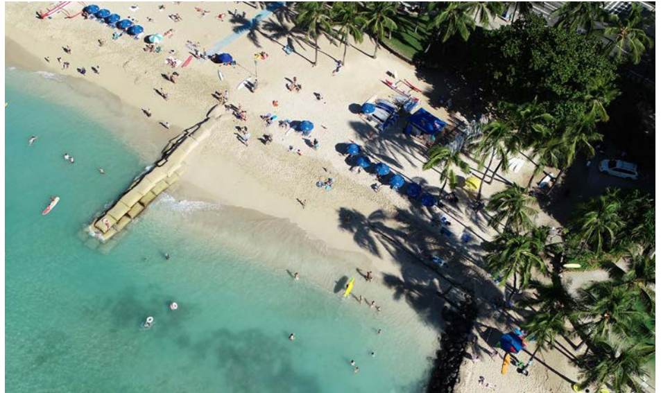
Kuhio sand bag groin (December, 2019). This project is a temporary fix to stabilize the area on the Diamond Head side of the sandbag groin.
